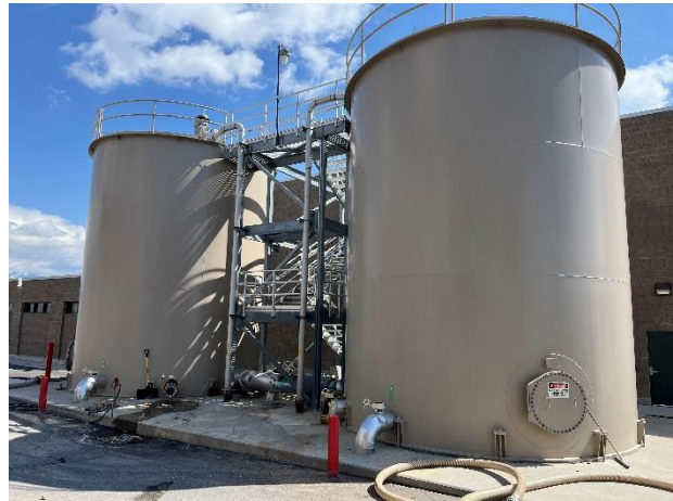
Figure 11-41: Sludge Blending Tanks
