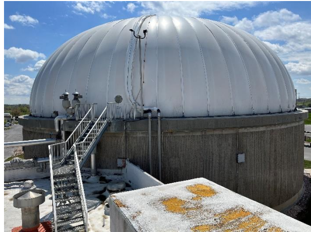
Figure 11-42: Secondary Digester No. 1
