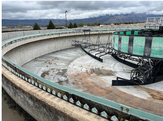
Figure 11-54: AS Secondary Clarifier with Repaired Floor
