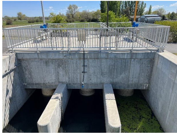
Figure 11-38: Final Effluent Pump Station
