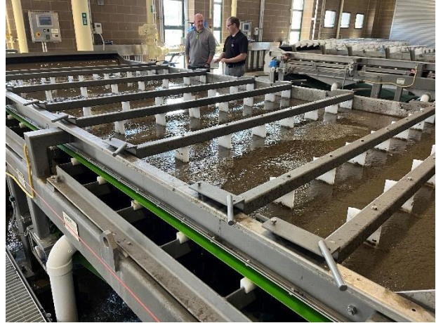
Figure 11-39: Gravity Belt Thickener
