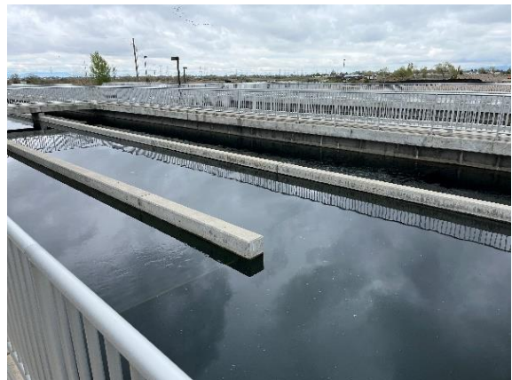
Figure 11-21: Chlorine Contact Basin
