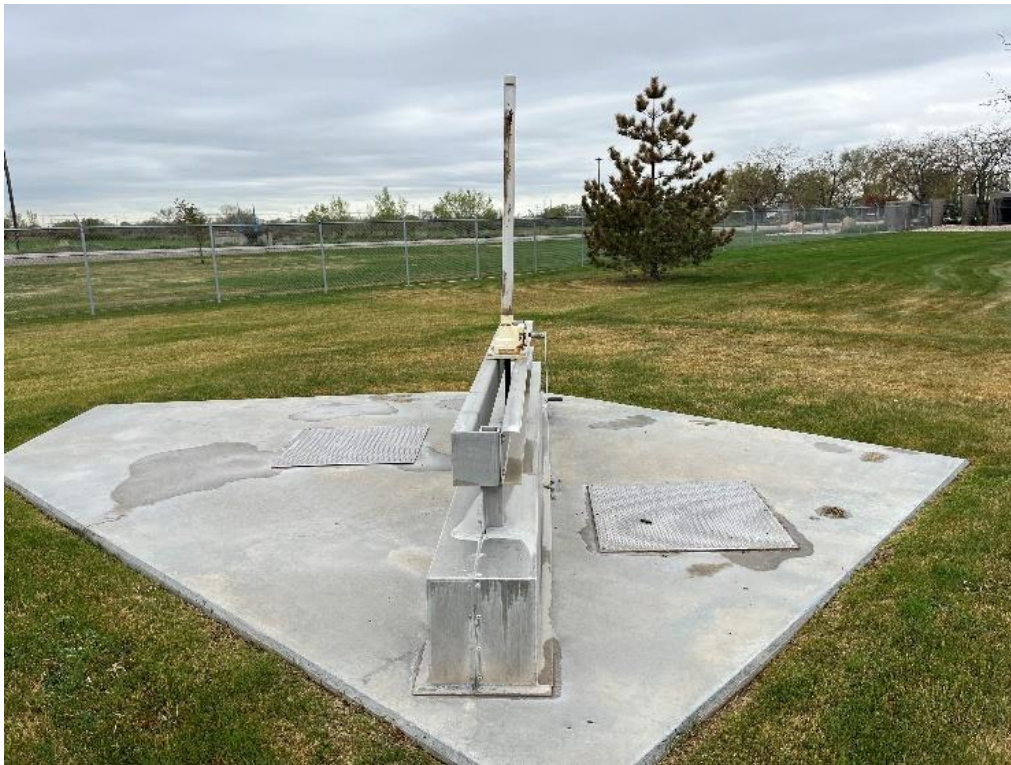
Figure 11-3: Headworks Influent Junction Structure
