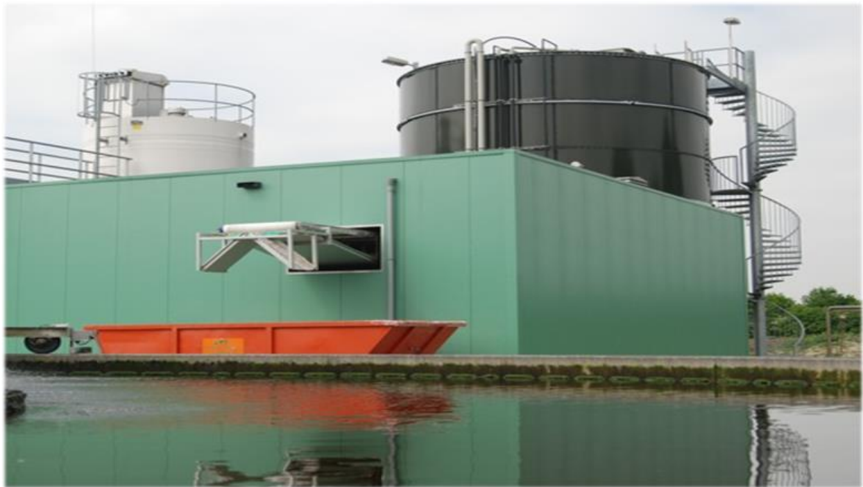
Figure:1 PHOSPAQ™ setup at Lomm, The Netherland (275 lds P/day)
