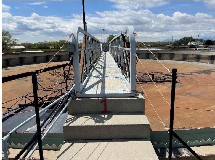
Figure 11-49: TF Primary Clarifier Handrail and Access Bridge
