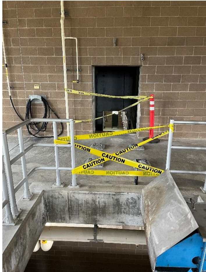
Figure 11-51: In-House Project to Remove Serpentix™ Open Conveyor
